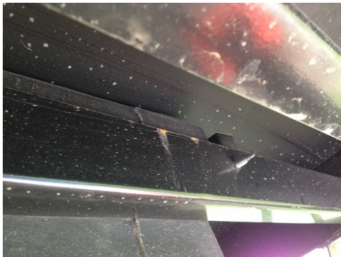
Rust on a black tank cross-member.
