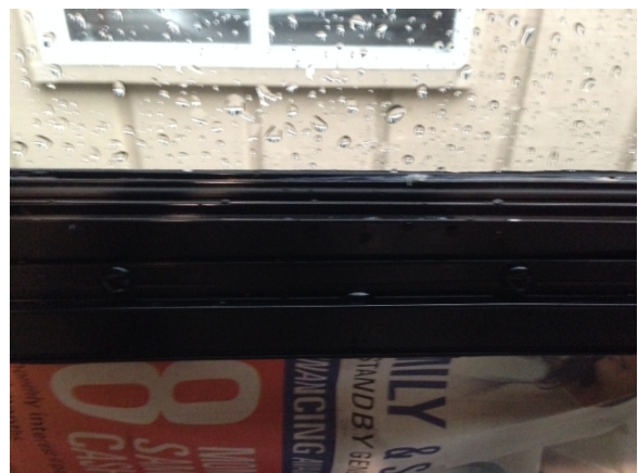
Photo 1: Kitchen Window, outside left taken this morning before I resealed it with Dynaflex 230.
